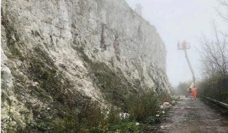
Given the evidence of instability in the cliff face, and its heavily overgrown nature in places, an assessment was required, along with stabilisation measures to ensure the safety of members of the public using footpath.
