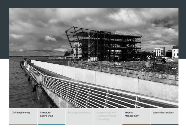
Alan Wood & Partners assisted Wykeland Group Ltd (in conjunction with the Environment Agency) in constructing a new section of flood wall to provide protection to the City of Hull and secure a new site for development.
