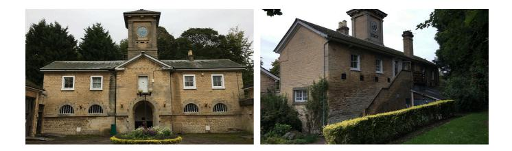
The building comprises traditional construction with Ashlar stone facework secured to the inner stonework with iron or wrought iron clamps. The roof is a mixture of pitched and flat roofs with slate and lead roof coverings, supported on a timber rafter and purlin roof structure. A feature timber roof light called the East Lantern was in place which allowed natural light into a two-storey atrium and stair area.
